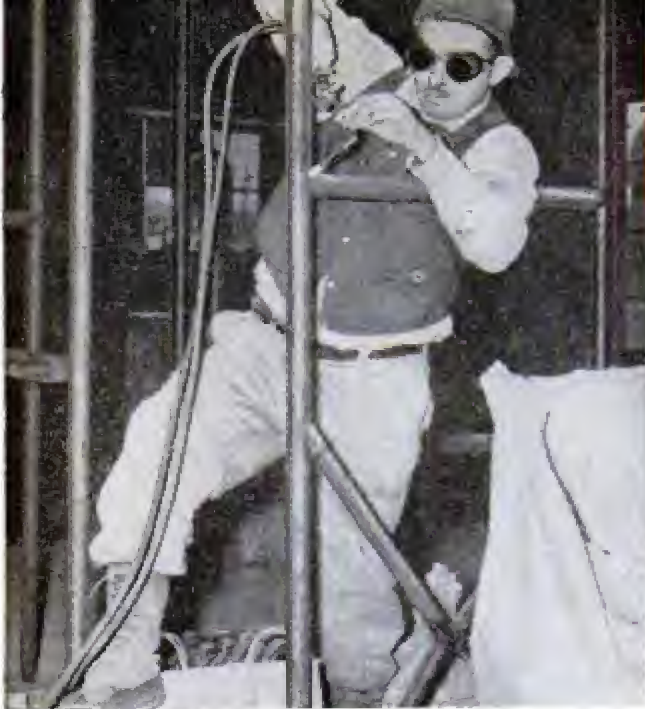
John F. Wagner of Johnstown, Pa., designer and builder of "pipe dream" house, uses steel pipes as both structural members and part of heating system
